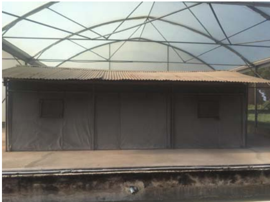
Fig. 1b: Exterior of the experimental hut built inside the SFS
